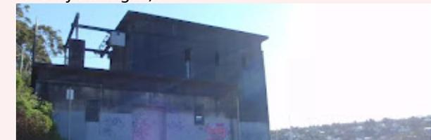
The Spit Syphon was built between 1922 and 1925 by the Public Works Department. It was necessary in order to pump sewage from the north without interfering with water transport. The building is styled with Egyptian influences as displayed by its tall, square concrete walls.
