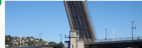
The Spit Bridge was originally built in 1924 to replace the punt service. The current Spit Bridge was built during the 1950's. The bridge is a bascule bridge, as it's middle section can be raised to allow tall ships through. This ability of the bridge does, however, stop traffic on a major arterial road, which has caused the bridge to be the centre of some controversy. The Spit Bridge carries the Spit Rd and the Manly Scenic Walkway.
